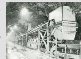
Mitsuboshi conveyor belt installed in the Omachi Tunnel of the Kurobe No. 4 Dam
